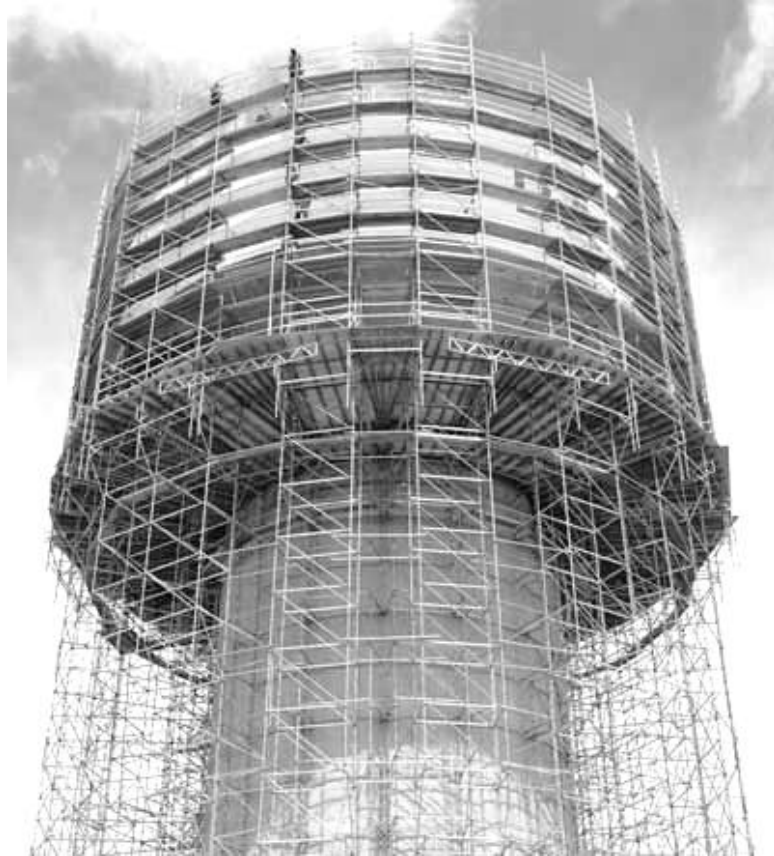
Figure 7.7(a) Tubular scaffolding
